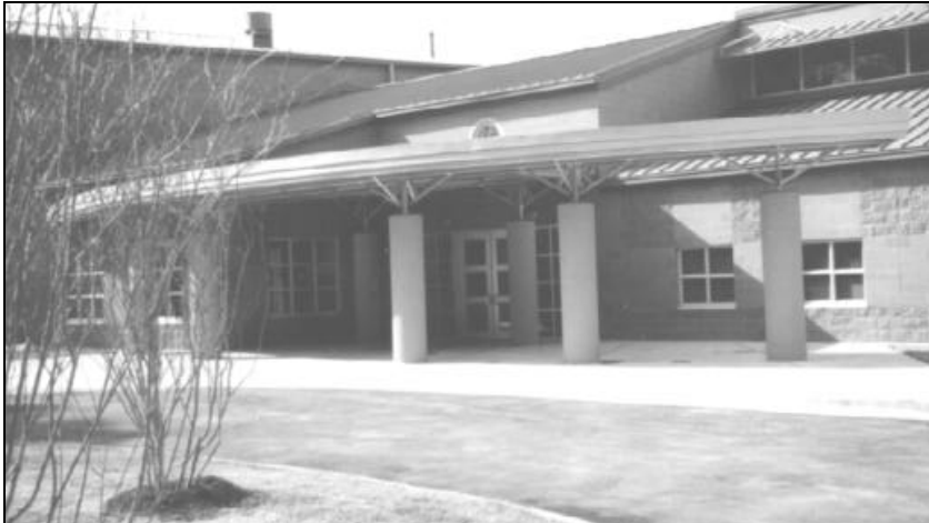
Dalton Whetstone Boys & Girls Club's dramatic canopied entrance awaits the flood of eager southwest Little Rock kids.
